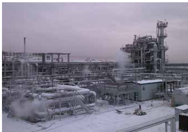
Extension of Yuzhno-Balykyskiy Gas Processing Complex - courtesy of Promstroj Group
