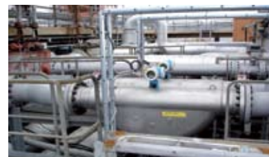
Modern inlet mass meters used for physical applications
